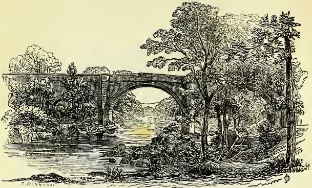
KIRKBY LONSDALE BRIDGE.—NORTH VIEW.
